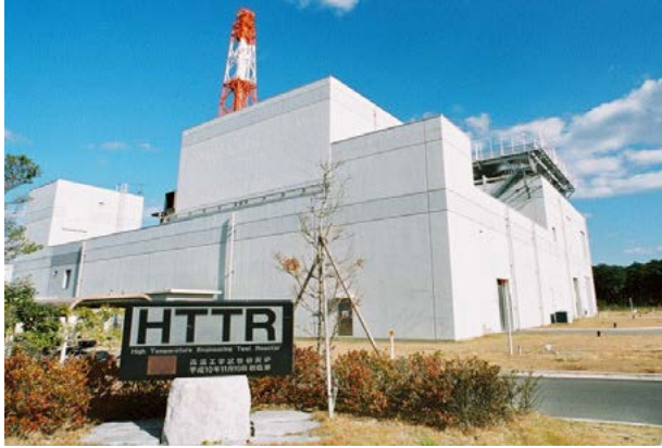
Fot. 1. The building of the HTTR reactor (photo: JAERI)
